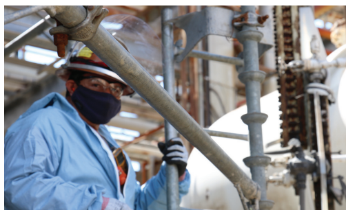
A contractor employee inspects equipment prior to the start of the Rock Dat Turnaround.
