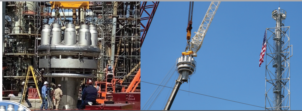
An innovative flare tip is now in place in Norco's OL-5 Olefins Unit. Designed to minimize smoke and noise during necessary flaring, the 20,000 pound tip was carefully lifted from the ground to its 300 feet high position in the OL-5 Unit during the site's recent turnaround. External Relations Manager Rochelle Touchard , at left, rode in a crane basket to take a close-up look at the new tip just days after it was positioned - and before the unit was back online.
