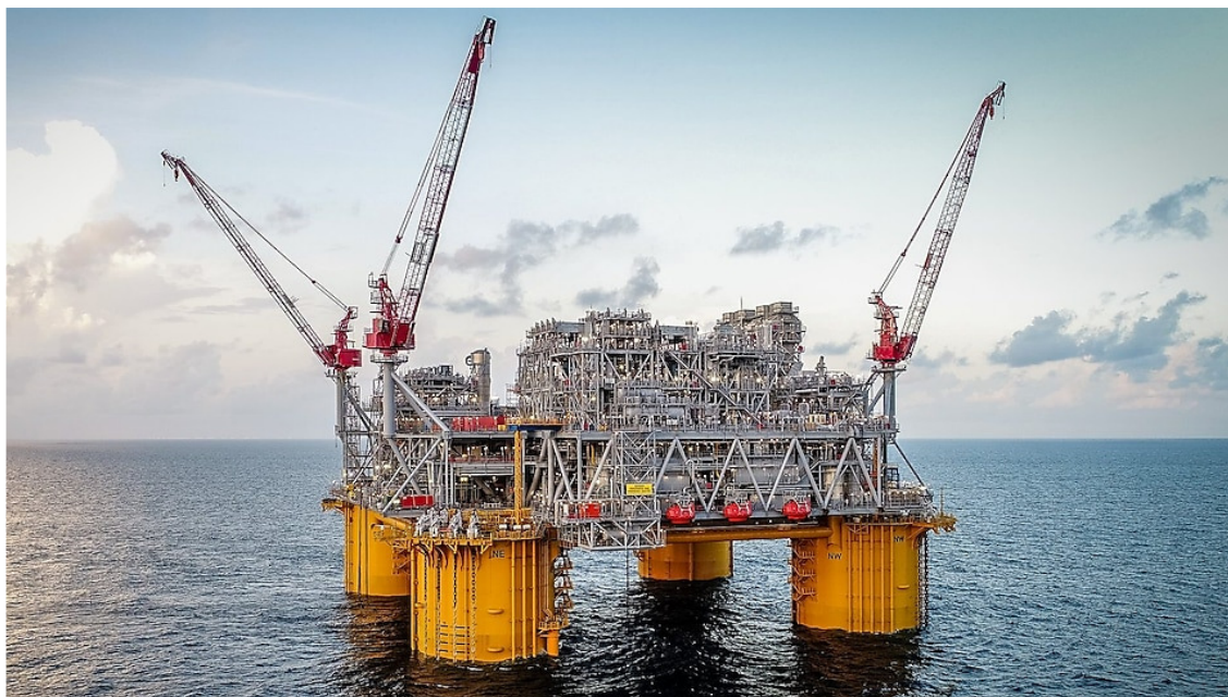
Shell's Appomattox Platform in the Gulf of Mexico
